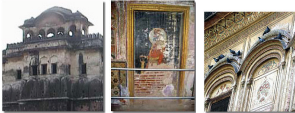
1. Qila Mubarak, Patiala - outer walls 2. Qila Androon, Patiala - damaged fresco 3. Qila Androon, Patiala - pigeon damage on walls
